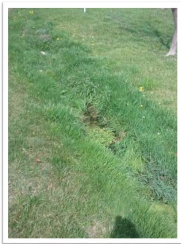
“Close-up” of ditch where a sewage smell was reported.
